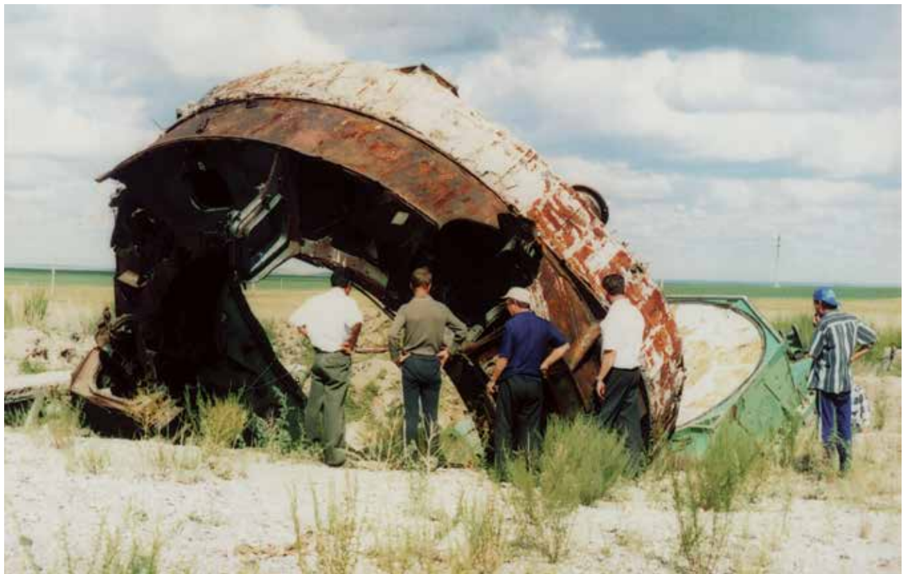
Ukrainian workers at SS-19 launcher silo complex
