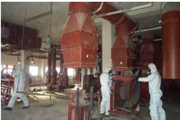
Workers destroying Stepnogorsk BW Production Complex
